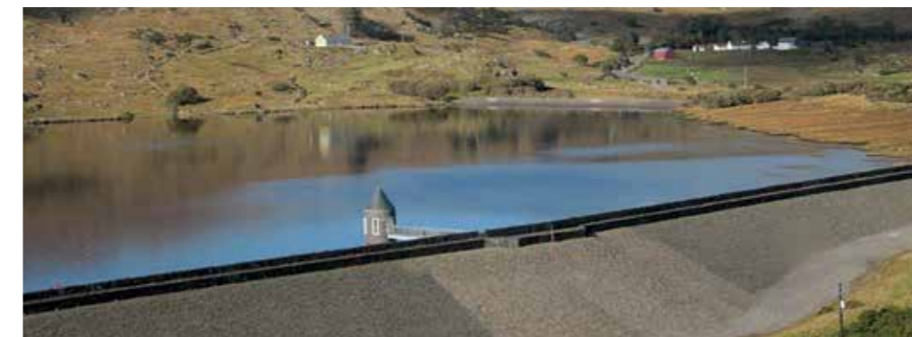
The dam which powers the hydroelectric plant at Island Seafoods, Killybegs, Co. Donegal
